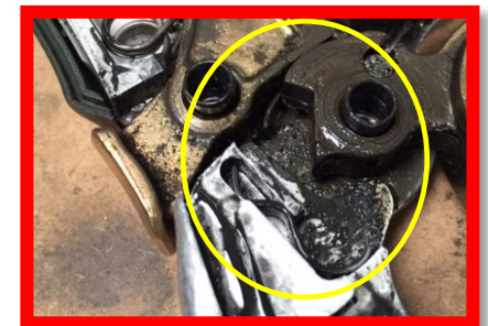
SPRING OF U-HOOK BROKEN
